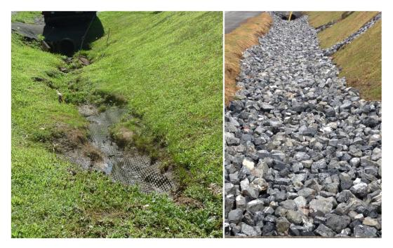
Swale carrying a large amount of runoff down a relatively steep slope had been protected by a nylon mesh, however it proved insufficient to prevent the erosion. Addition of rip-rap to the swale to protect it from erosion has worked well and the erosion has not returned.
