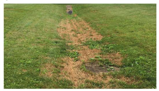
Shallow swale with a low slope. Water apparently ponds in part of the swale, damaging the grass which is not water tolerant. This can probably be fixed by reseeding with a grass that is more tolerant of wet conditions. Allowing the grass to grow taller (6-12" after mowing) will promote stronger root systems, and increase transpiration (the water a plant releases into the air) helping the soil to dry out between storms.
