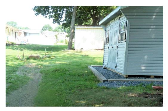
This is a shallow swale in an older development. During storms it carries a high volume of stormwater resulting in erosion problems. Because of the shallow side-slopes, it can become very wide during storms. Obstructions to the flow, such as this shed, should not be placed in or near a stormwater conveyance because of the potential of water damage to the shed and contents, and also because an obstruction can raise the flood elevation elsewhere causing further damage.
