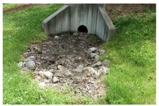
Rip-rap at an endwall that has become clogged with sediment. The purpose of the rip-rap is to slow the flow through the swale. Reduced flow velocities decrease the chance of erosion. When rip-rap becomes clogged with sediment, it can no longer function to slow flow rates and should either be cleaned out or replaced.
