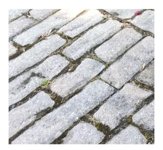
Paving stones with soil filled gaps between the stones. For this surface to be permeable, the soil in the narrow gaps must be highly permeable. Stone is usually used in the gaps because of its higher permeability.
