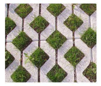
Pavers with larger soil-filled gaps planted in grass. This surface is more permeable than the one above, however with the grass present it is not suitable for high-traffic areas.
