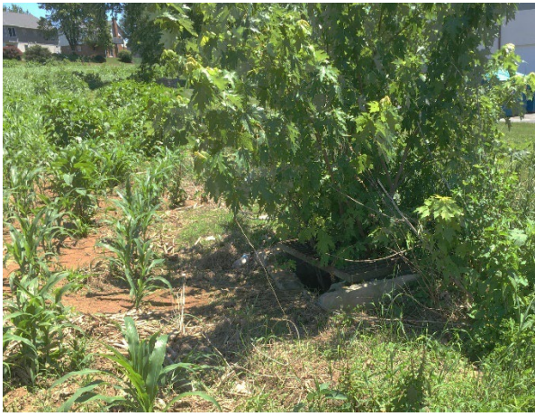
A long-neglected inlet with a maple tree growing up through the grate. The concrete around the grate has also broken up.
