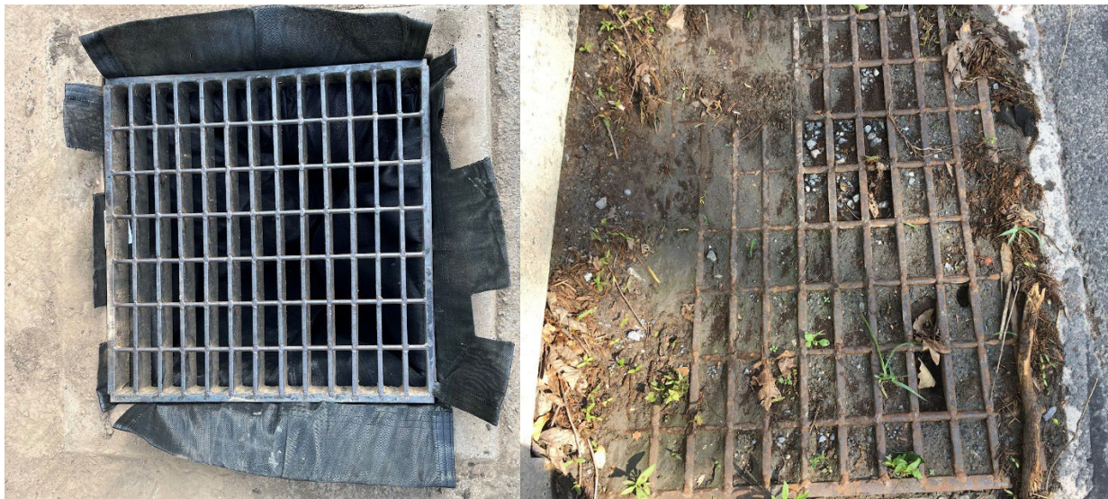
Inlet with filter bag in good condition.
