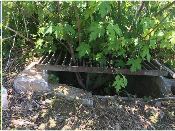
A long-neglected inlet with a maple tree growing up through the grate. The concrete around the grate has also broken up.
