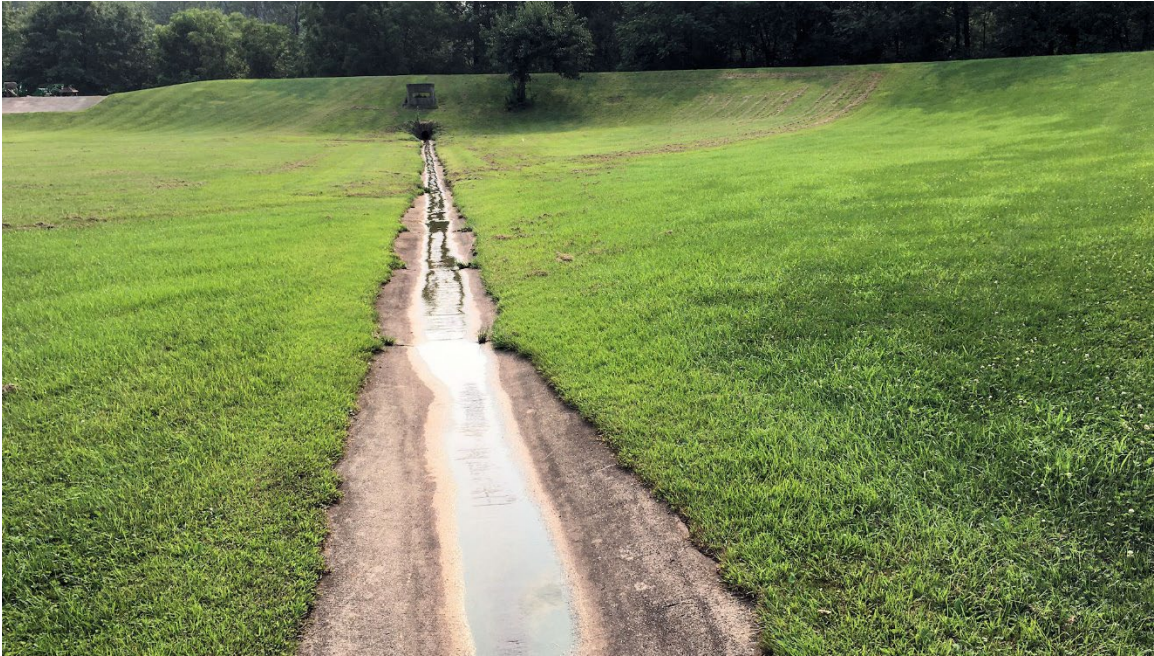
A concrete lined low-flow channel can prevent erosion.
