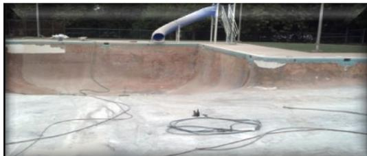
*The water blasting process has started as well as plastering of pool floor.*
